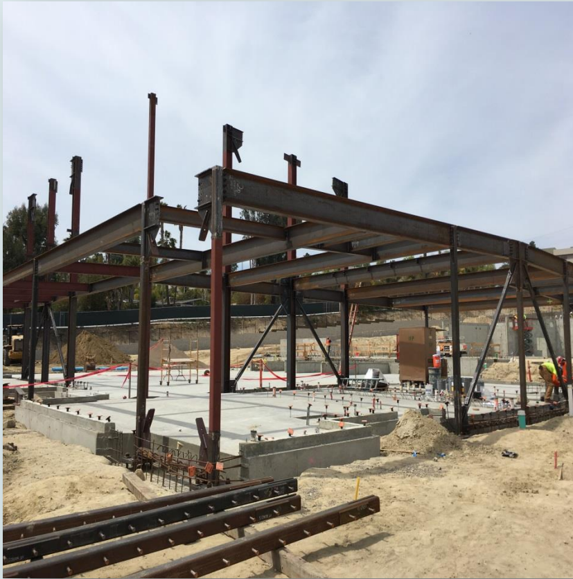
EWMS Campus Re-Construction
