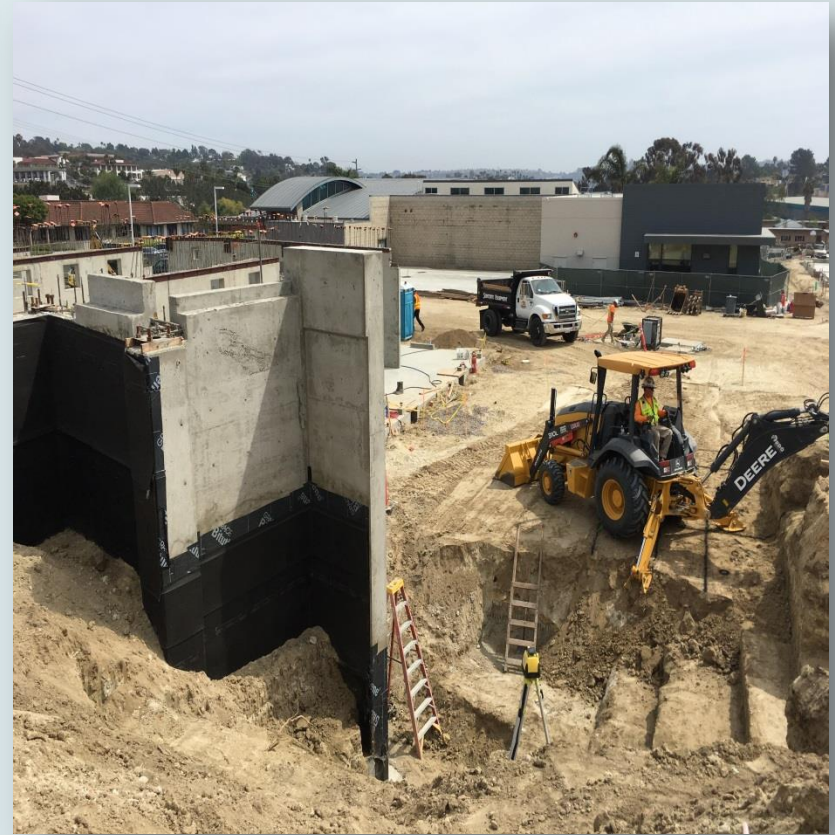
EWMS Campus Re-Construction
